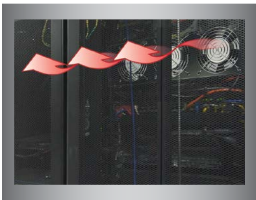
Active heat removal uses fans attached inside the enclosure to pull heat up and out of the cabinet.
